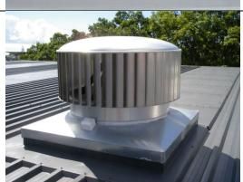
6 Issue: Condensation Drip (after hours) for ventilator with damper.
