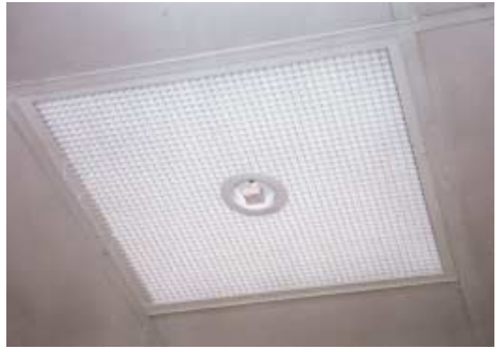
EC Damper Grille is made of corrosion resistant aluminium in a powdercoat finish.
